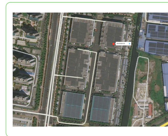
Solar Photovoltaic Panels on the Roof of SUNMI Manufacturing Plant
